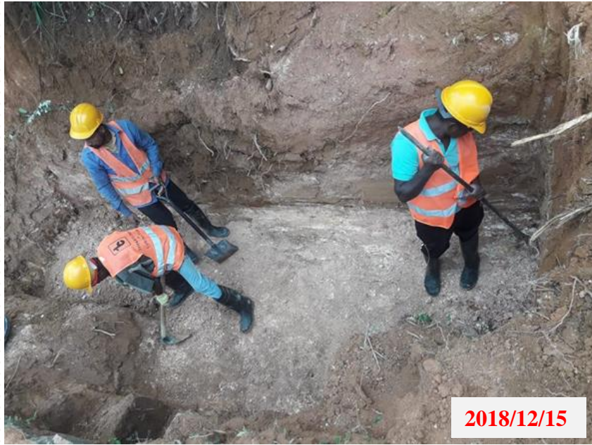
Preparation of Culvert Screed Bed UBA-76 CH. 1+189
