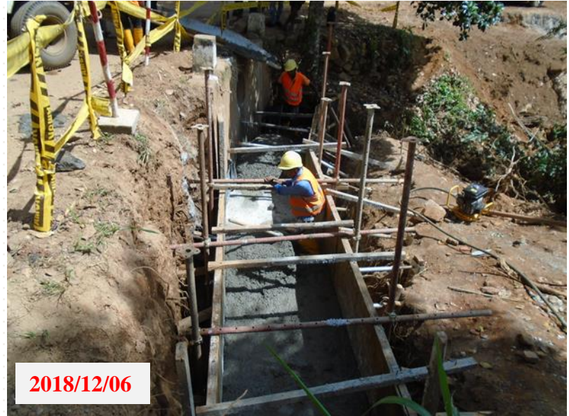
Culvert Base concreting at UMO-110 CH.12+070(RHS)
