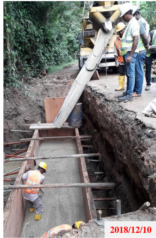
Head Wall 1st step Concreting UMO-47 at CH. 1+406 (RHS)
