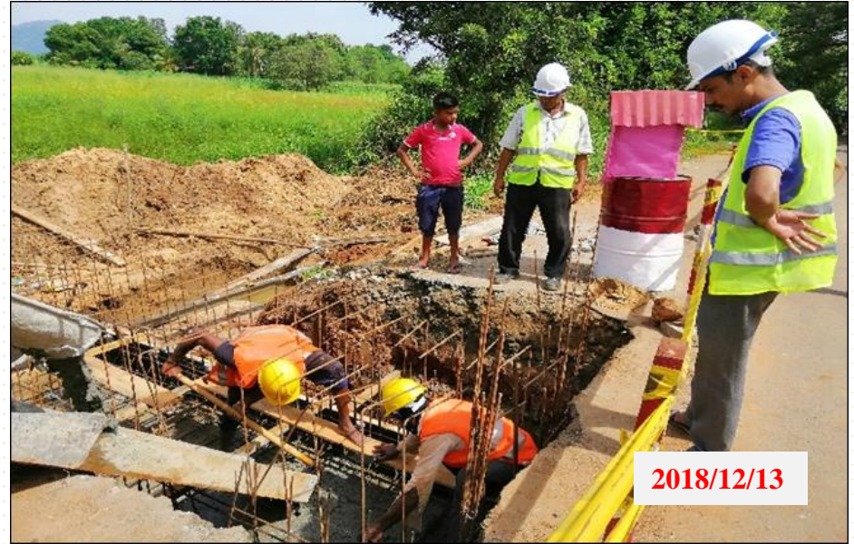
Culvert construction UMO-059 CH.7+186 (RHS)
