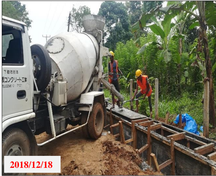
Line Drain Construction UMO -059 CH.(8+950 RHS)
