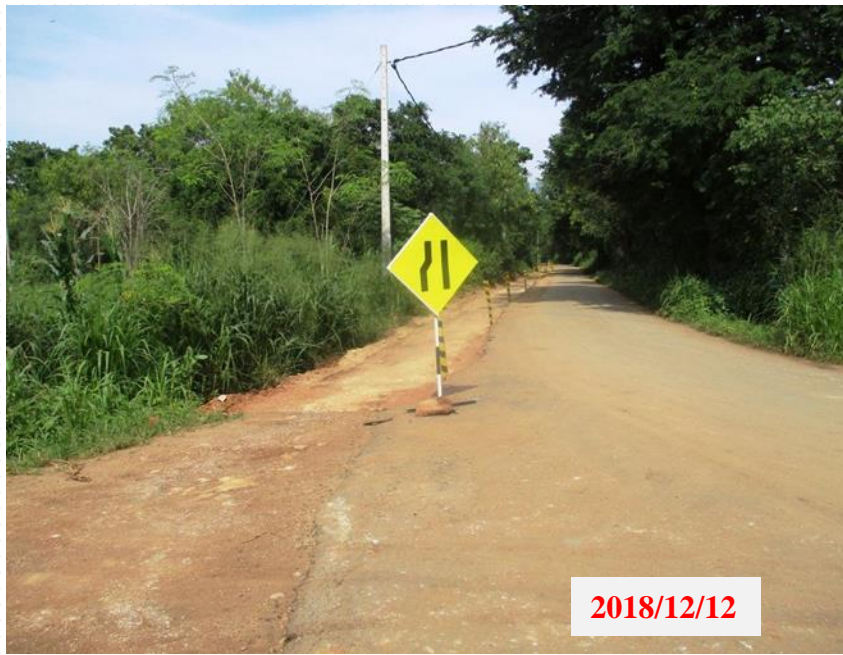
Embankment construction UMO 020 CH. 1+400 (LHS)
