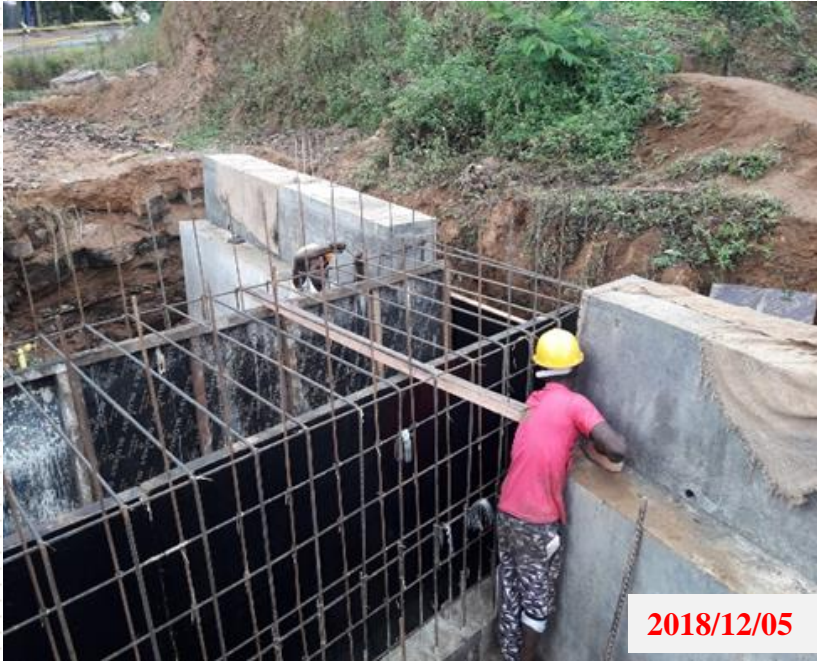
Box Culvert Reinforcement binding UBA-242 CH 4+208
