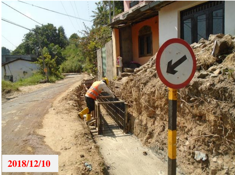
Line Drain Construction UBA 361 at Ch.0+420
