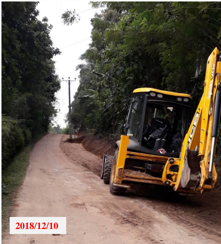
Road clearing and grabbing UMO-94 at Ch. 0+300 - 0+500 (RHS)
