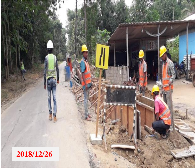
Form work for drain wall concreting in UMO-077 CH.0+300 (RHS)
