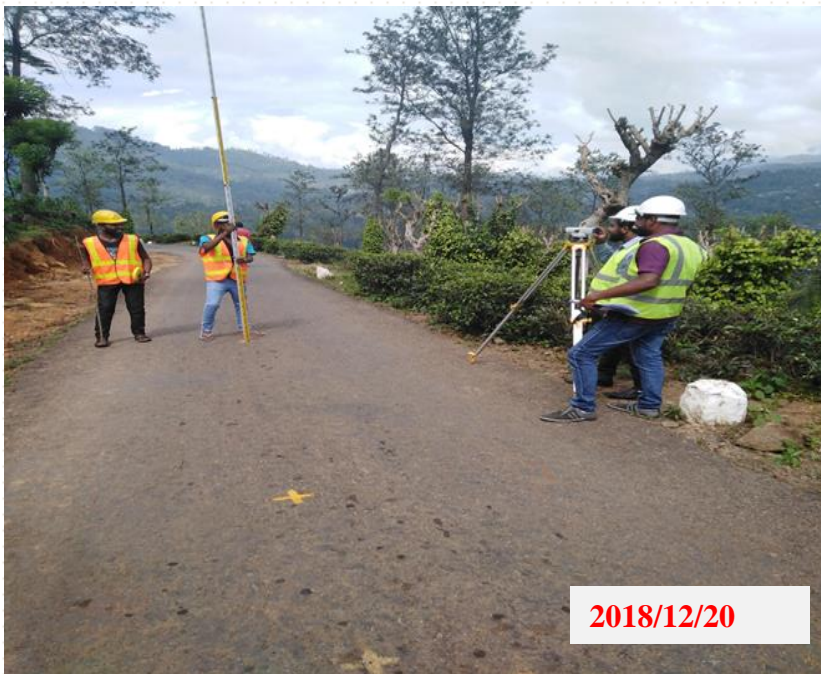
Taking Initial Cross sections UBA 341 CH. 1+000
