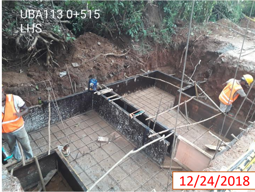
Culver abutment and H/W Base UBA113 CH. 0+515(LHS)
