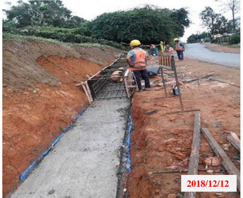
Formwork Preparation for Lined Drain UBA- 242 CH.4+652(RHS)
