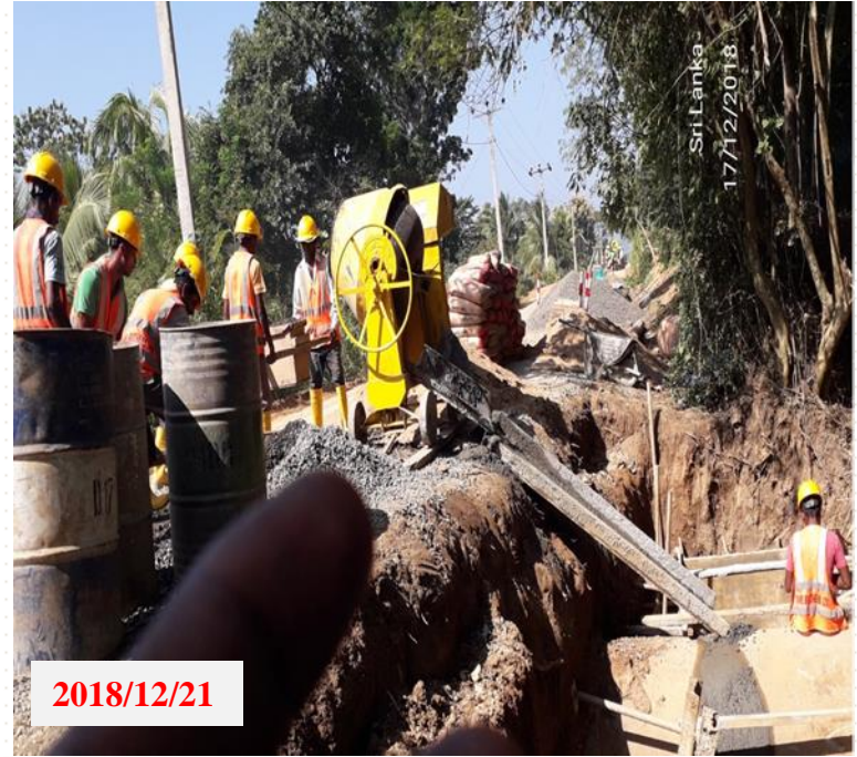
Culvert head wall concreting in UMO-077 CH.6+864 (LHS)
