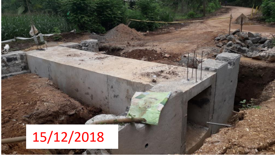
Reconstruction Box Culvert UBA-212 CH.1+387
