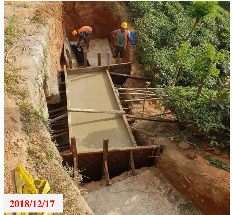
Concreting at Widening Culvert Road UBA-081 CH.5+410
