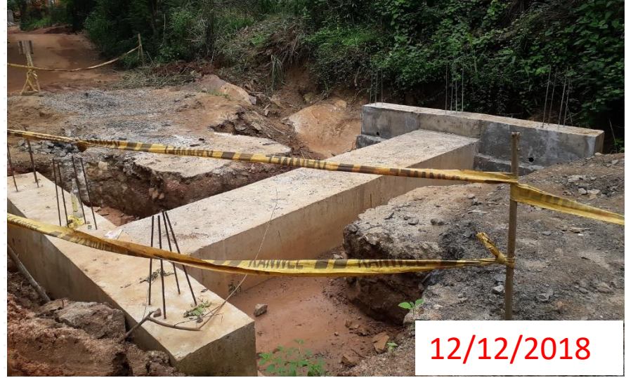
Reconstruction Pipe Culvert before backfilling UBA-212 CH 0+078
